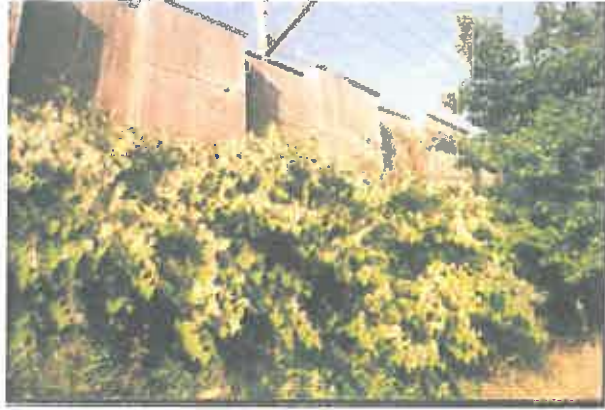
Plywood noise barrier
