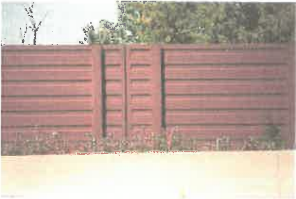
Metal noise barrier
