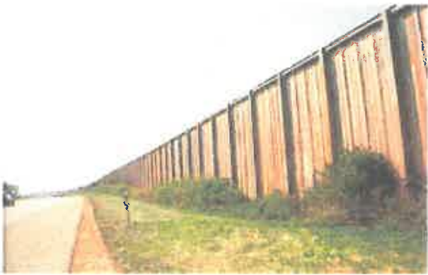
Glue laminated post and plank noise barrier
